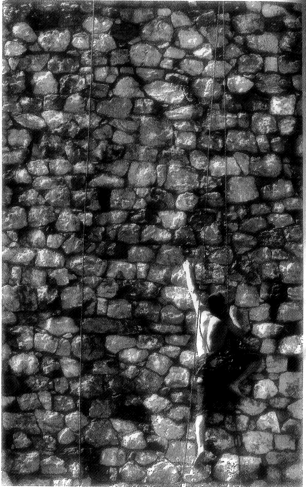
A man practicing climbing on a rock-wall building. Source: istock.
